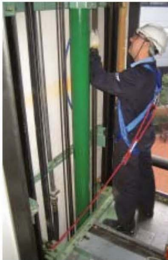
Engineer standing upright showing lanyard taut
