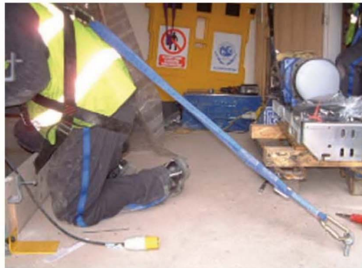
Engineer kneeling down next to hoistway opening with lanyard taut
